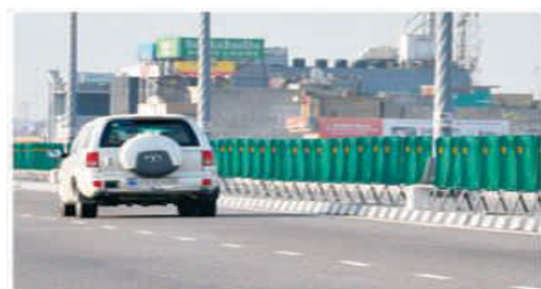
Typical Installation of Anti-Glare Screens on the Median
