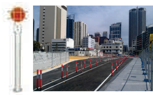
Solar Delineator with Guide Posts and their Typical Installation
