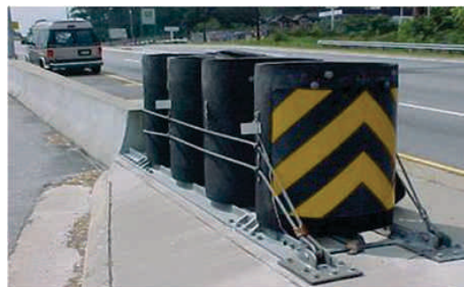
Typical Installation of Crash Cushions at the Gore Area
