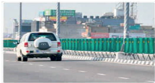
Typical Installation of Anti-Glare Screens on the Median
