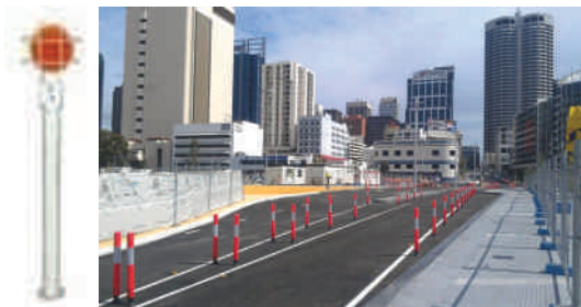
Solar Delineator with Guide Posts and their Typical Installation
