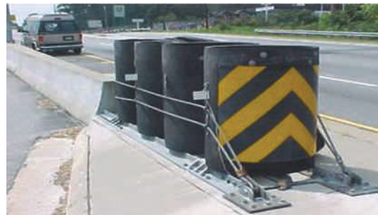
Typical Installation of Crash Cushions at the Gore Area
